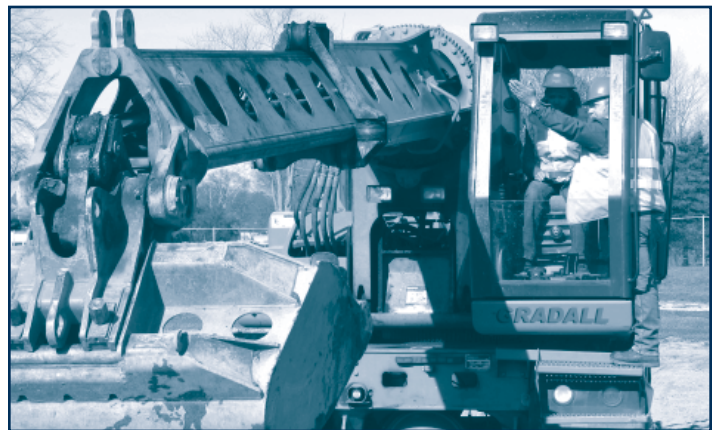
Terry Ream, a Heavy Equipment Operator from Ingham County Road Commission, helps a student use an articulating excavator.
