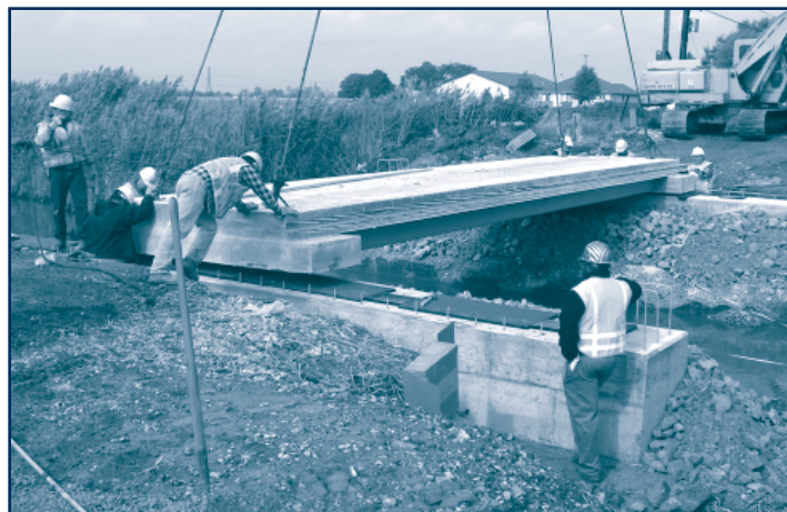
Monroe County Road Commission maintenance workers place a prefabricated deck slab for the new Suder Ave. Bridge.
